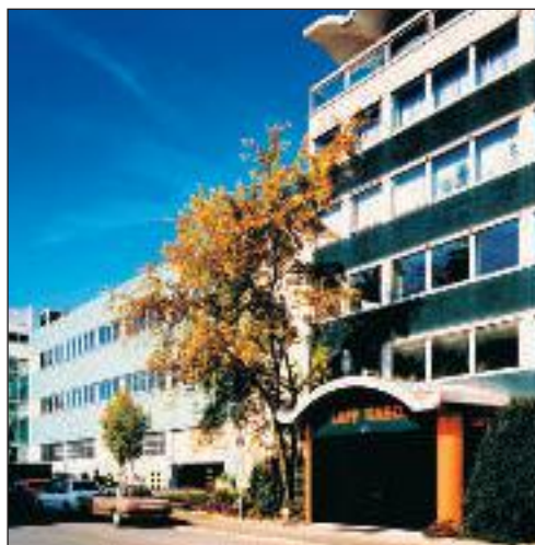
The Lapp Kabel headquarter in Stuttgart-Vaihingen.
